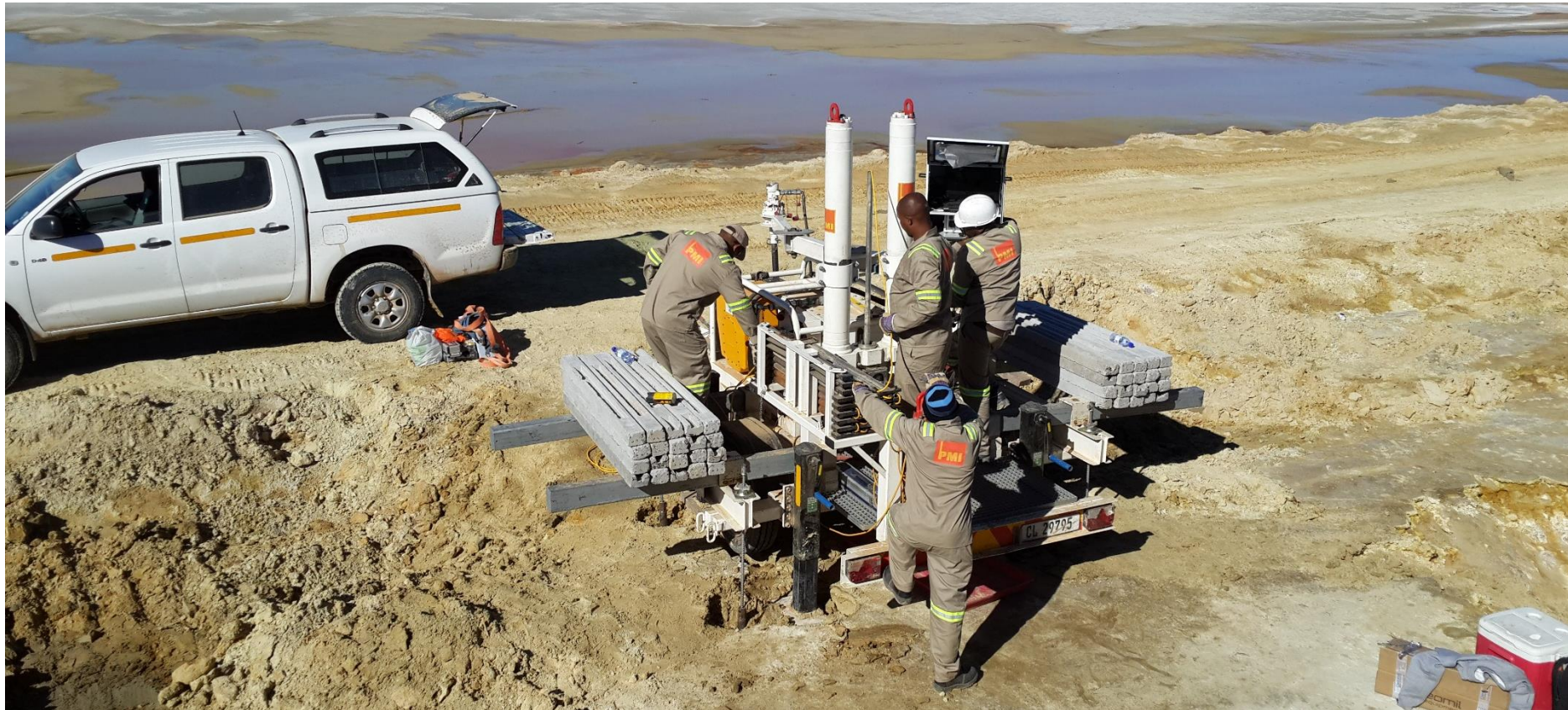
Ground anchors + dead weight
